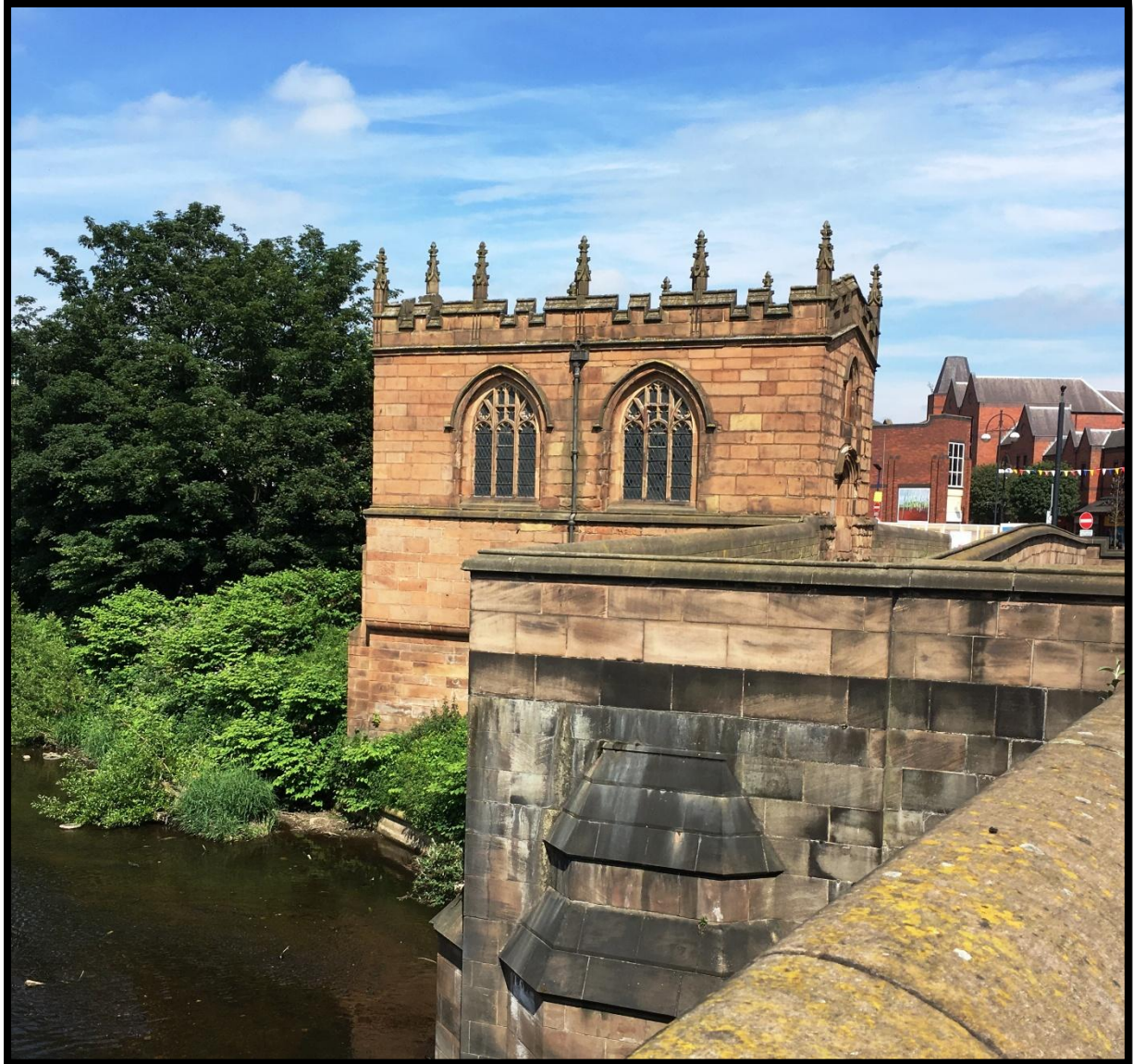
7 Rotherham Bridge Chapel
